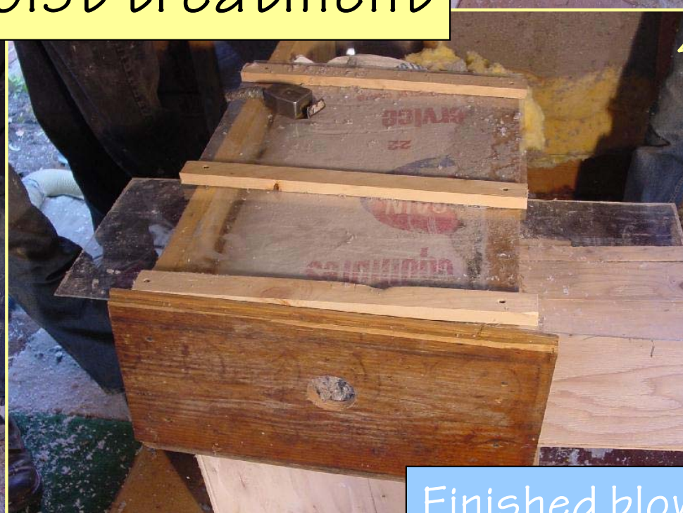
Open space blown with cellulose
