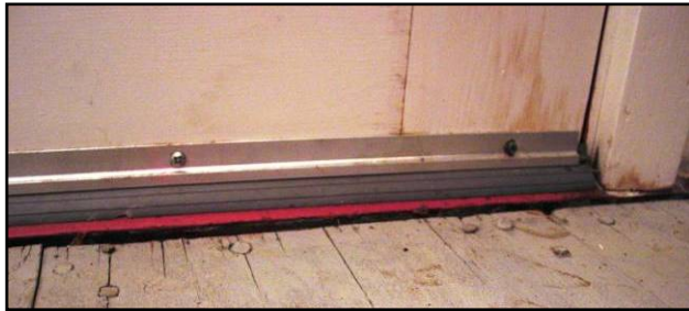
Exterior door threshold sweep
