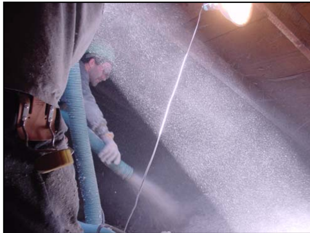
An open blow with cellulose in an attic
