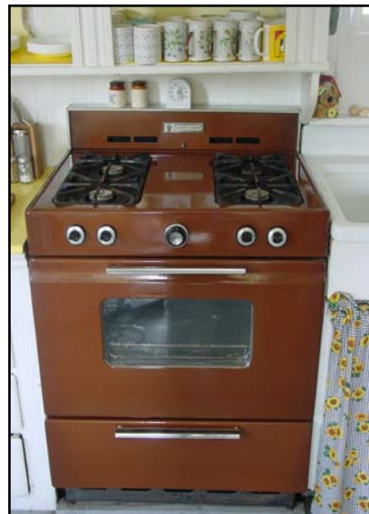
Kitchen range, four top burners, one oven bake burner
