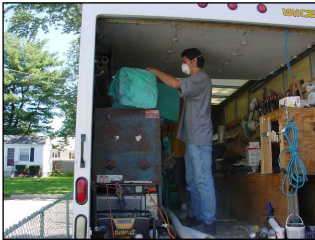
Filling the hopper of the Krendl insulation blowing machine
