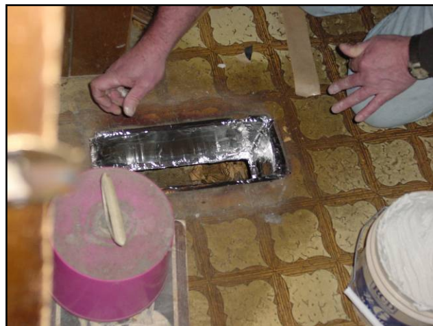
Using metal and mastic to seal mobile home duct boots
