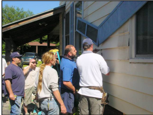
Knowledge of effective siding removal is very important
