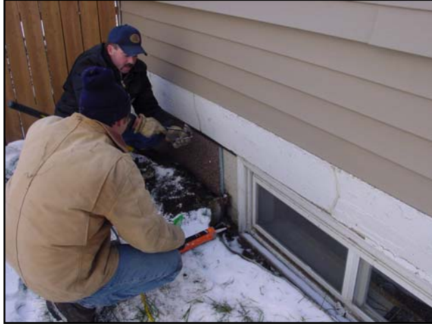
Installation of rigid exterior foundation insulation
