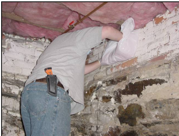
Stuffing the band joist area with an “insulation pillow” (a plastic bag filled with fiberglass)
