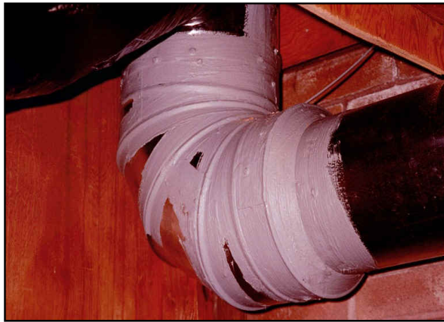
Use duct mastic to seal all ductwork in unconditioned spaces
