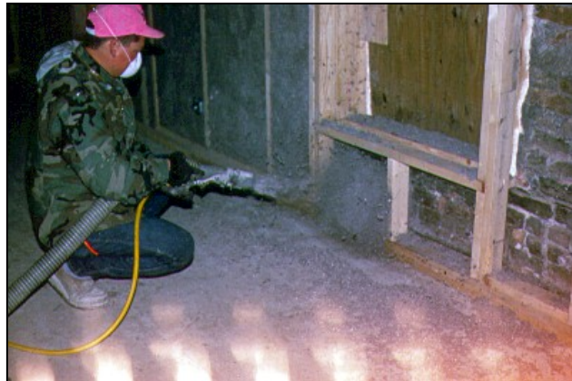
Wet spray cellulose being installed
