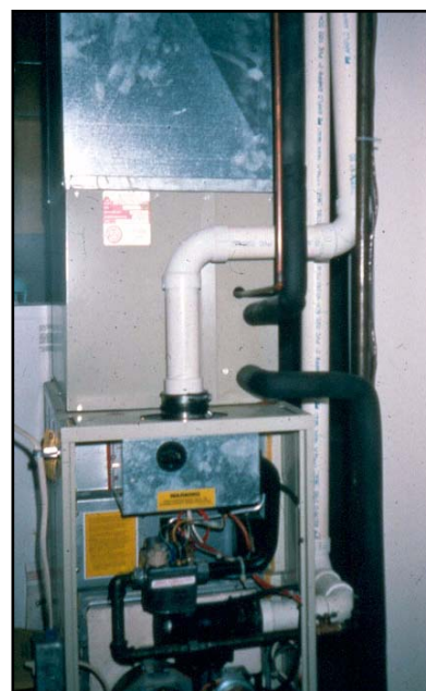
This direct-vent, sealed combustion gas furnace does not require worst-case draft testing
