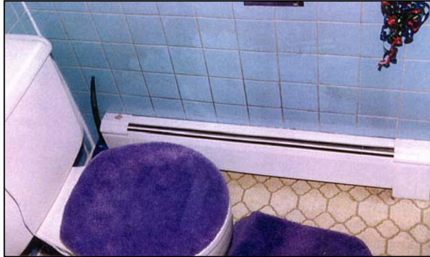
Hot water baseboard distribution usually operates with a maximum water temperature from 180 to 200°F
