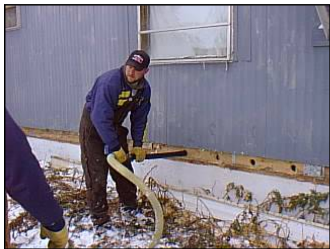
Blowing a mobile home floor
